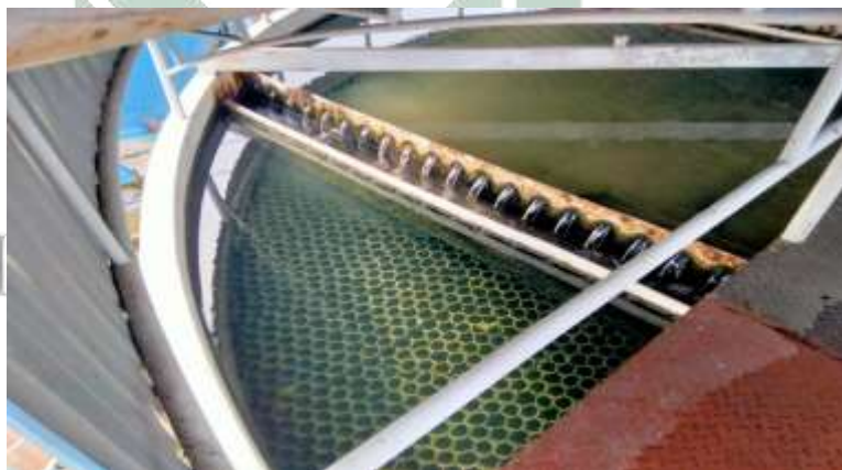
Gambar 4.11 Detail Gutter Dan Tube Settler
